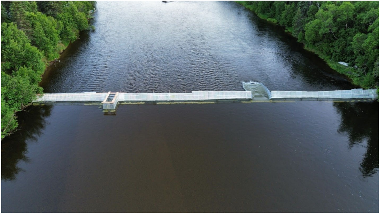
Photo 3. Overhead view of the Koktuli weir, showing livetramp (left) and floating panel boat gate (right), July 2024.
